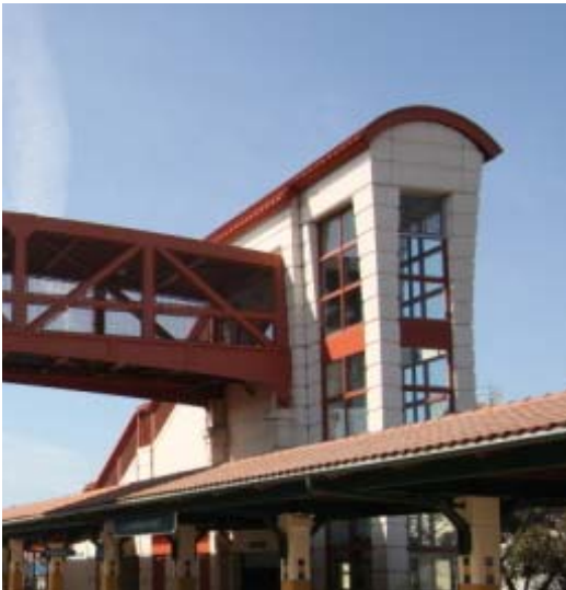
FIGURE 9.1 GLASS BACK ELEVATOR TOWER
